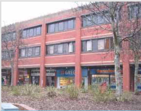
Units 1-5 Govan Cross Shopping Centre
